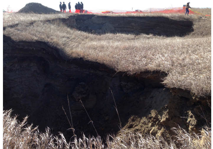
Large sinkholes caused by collapse of abandoned mine workings near Bowman
